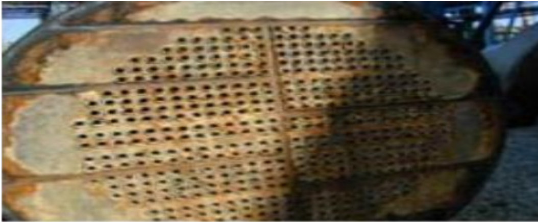
Fig. II.20 : Importante corrosion [18]
